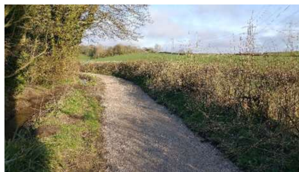
Snuff Mill Lane, resurfaced and flood-free
