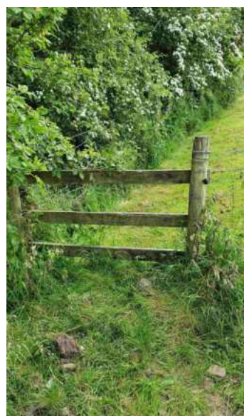
Stile with missing steps noted on a footpath check walk
