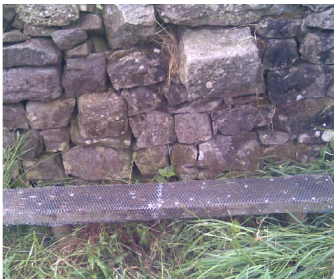
New wire netting on a step on Langthwaite Road
