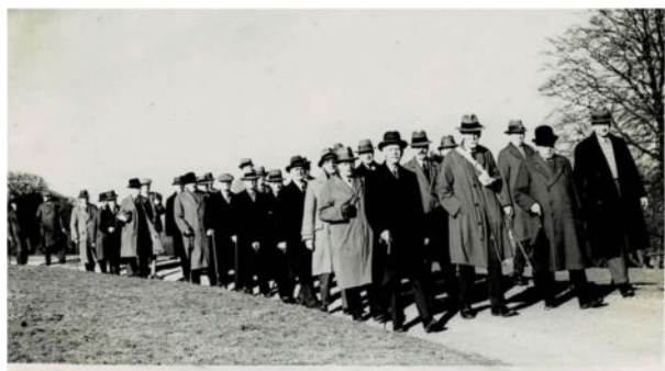
On the March Yealand Manor March 1 st 1939
